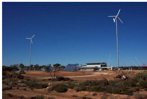
Figure 6: Westwind 10s installed.
