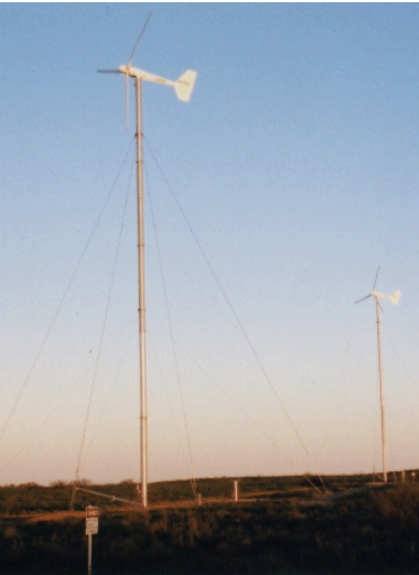
Figure 7: Westwind 20s installed.
