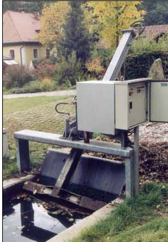
Figure 23 – Automatic intake screen cleaner.
