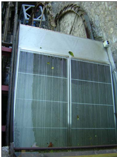
Figure 22 – A typical modern intake screen.
