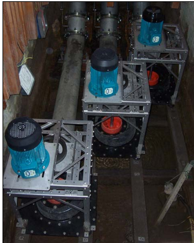
Figure 17 – 3 x Polymer Turbine installation. (Crabble Mill, Dover, Kent).
