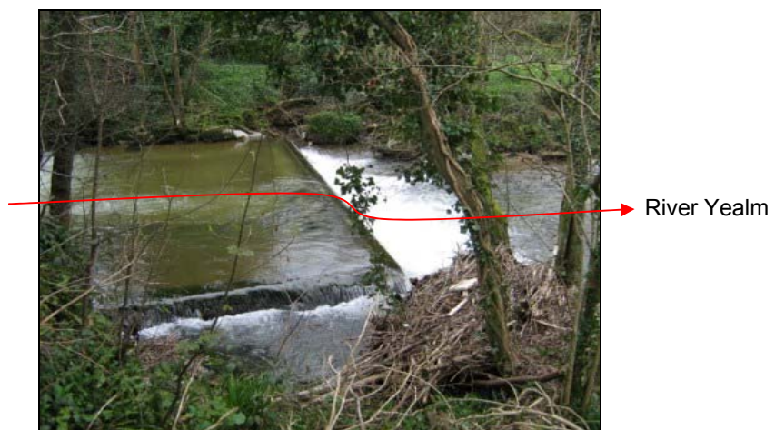
Figure 11 – Lowest step of weir, looking across weir structure.
