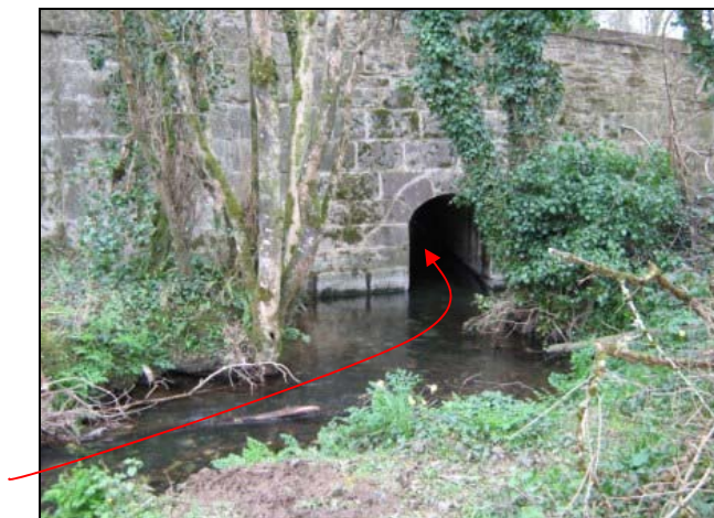
Figure 5 – Entrance to leat tunnel, looking downstream.
